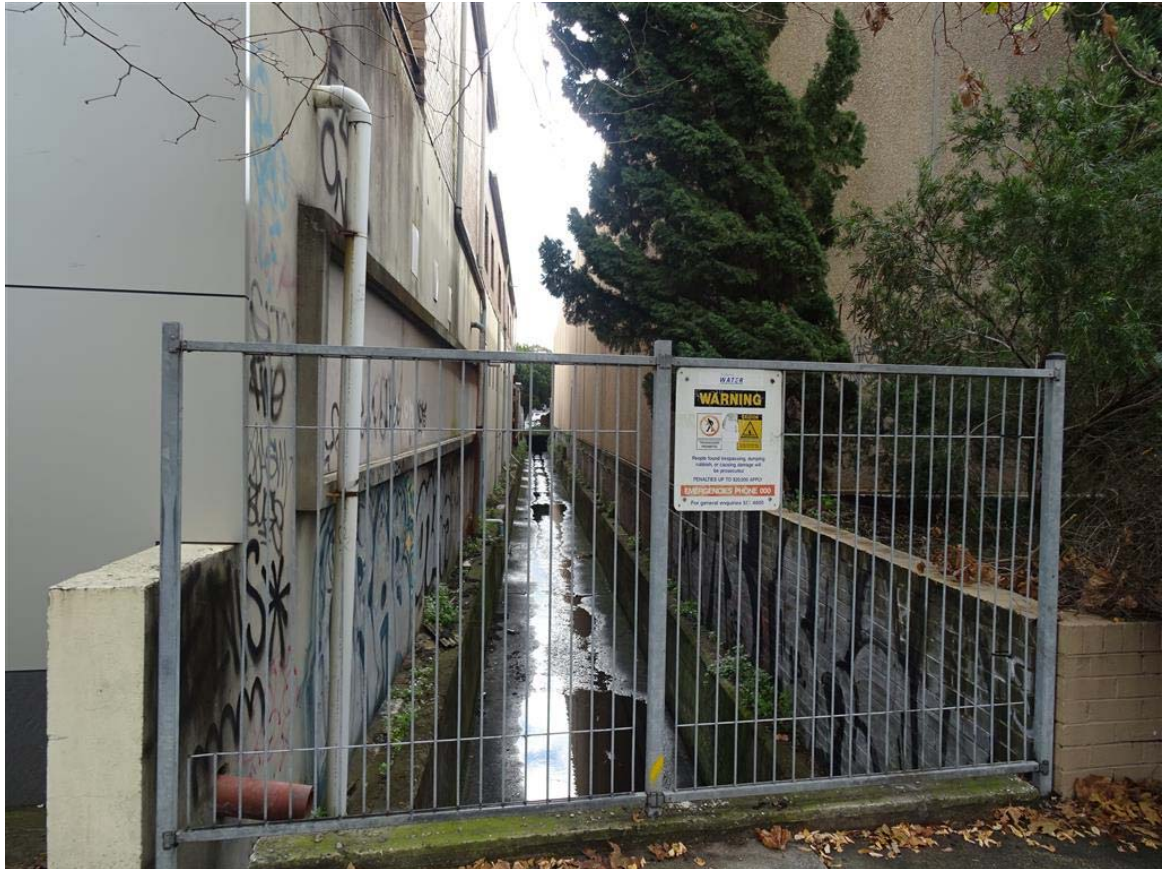
Figure 13: Neighbouring stormwater channel viewed from Botany Road.
