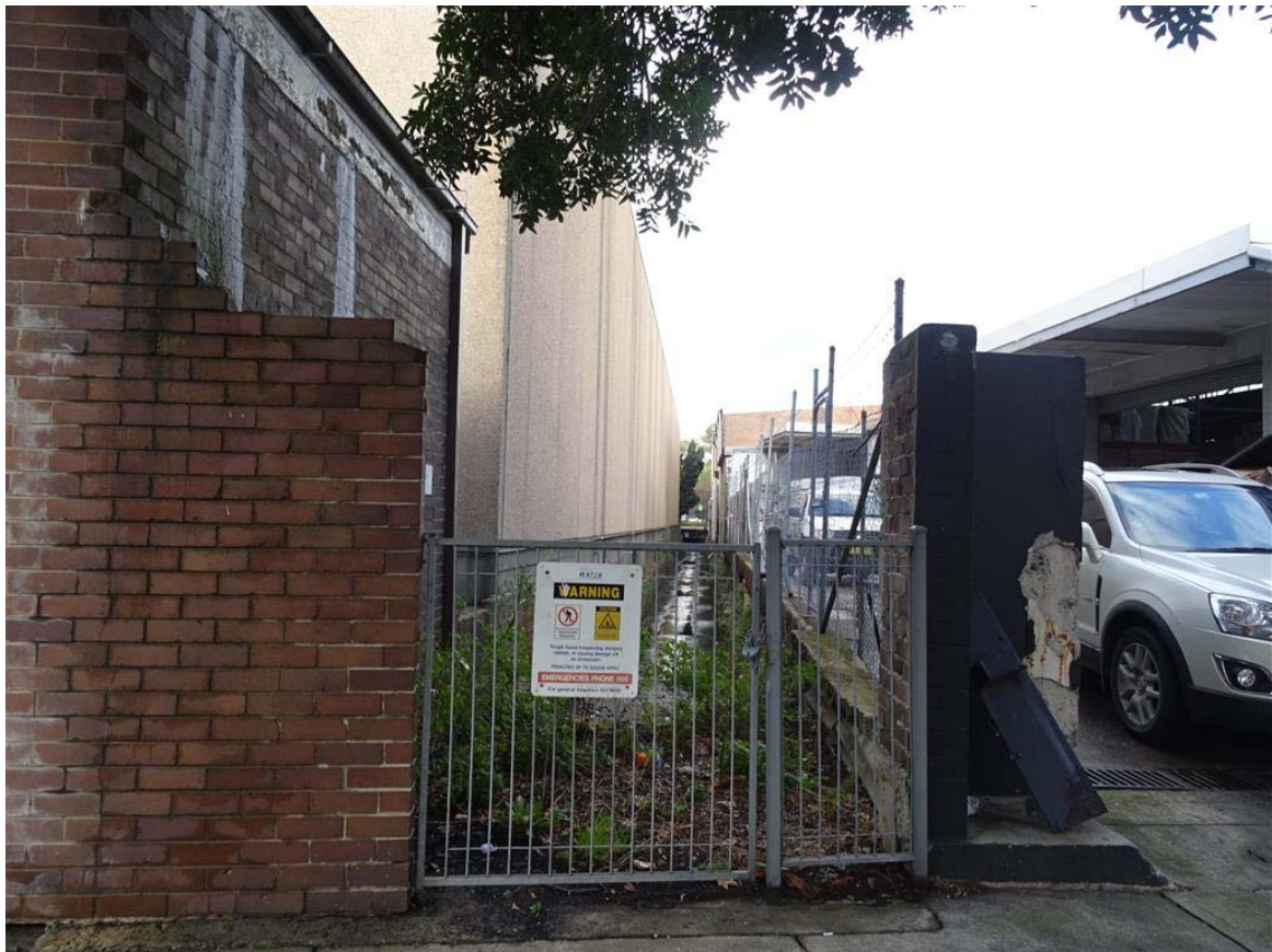
Figure 14: Neighbouring stormwater channel viewed from Ralph Street.
