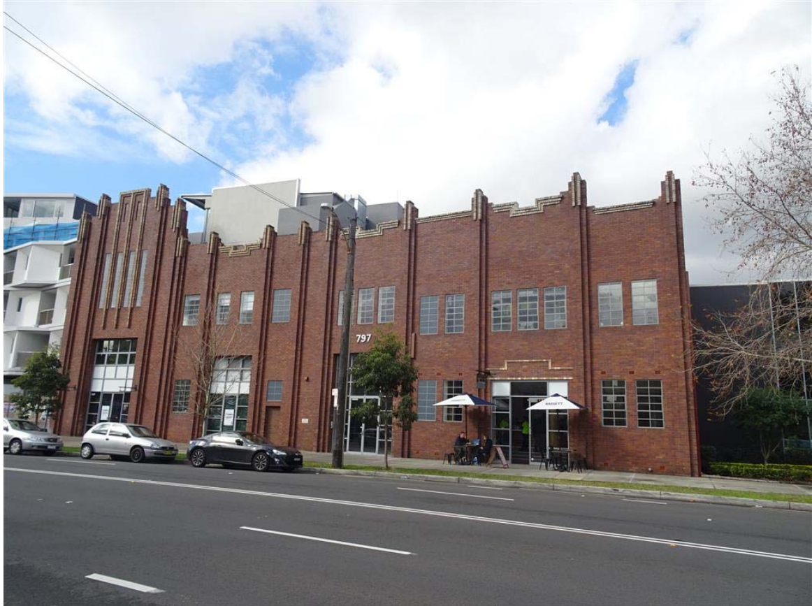
Figure 11: Existing heritage item on the opposite side of Botany Road.
